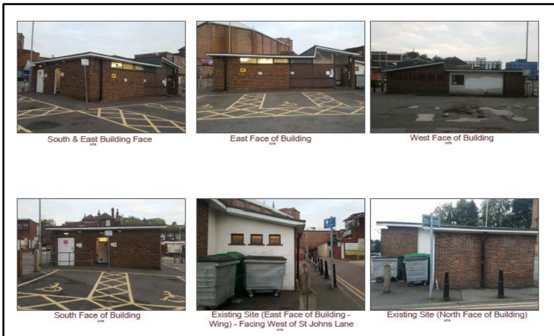
Figure 2 Photos of Existing Building
